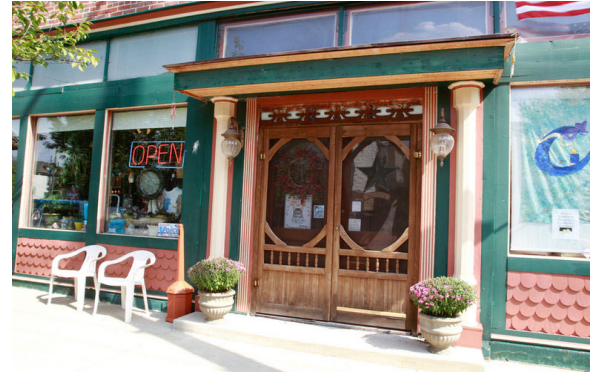
Transom windows above the storefront display
