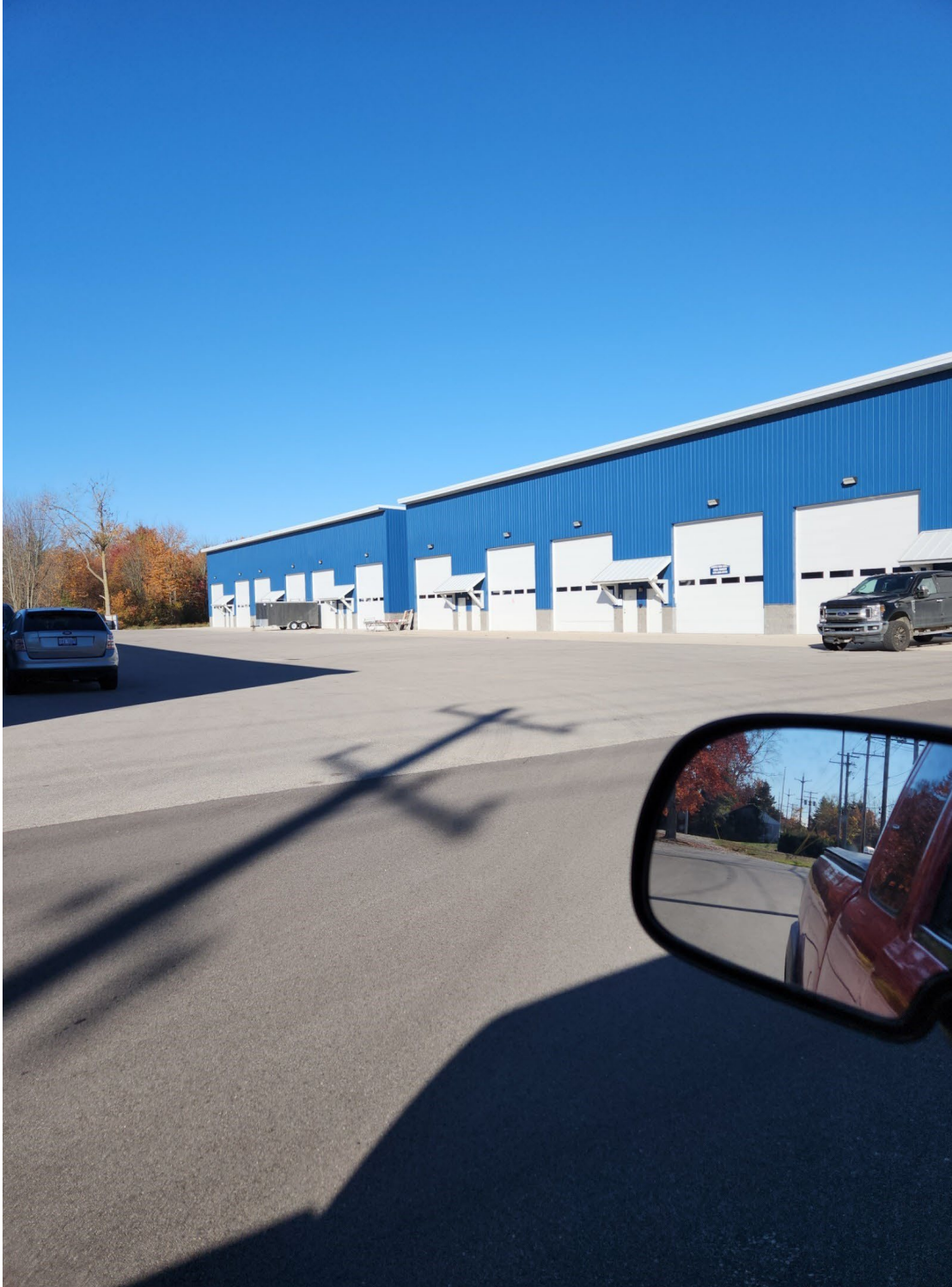
Overall site view and building access
