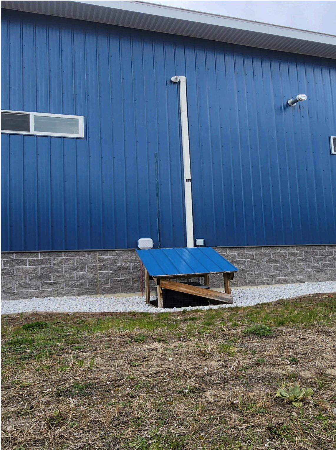
Rear drainage and future air-conditioning readiness
