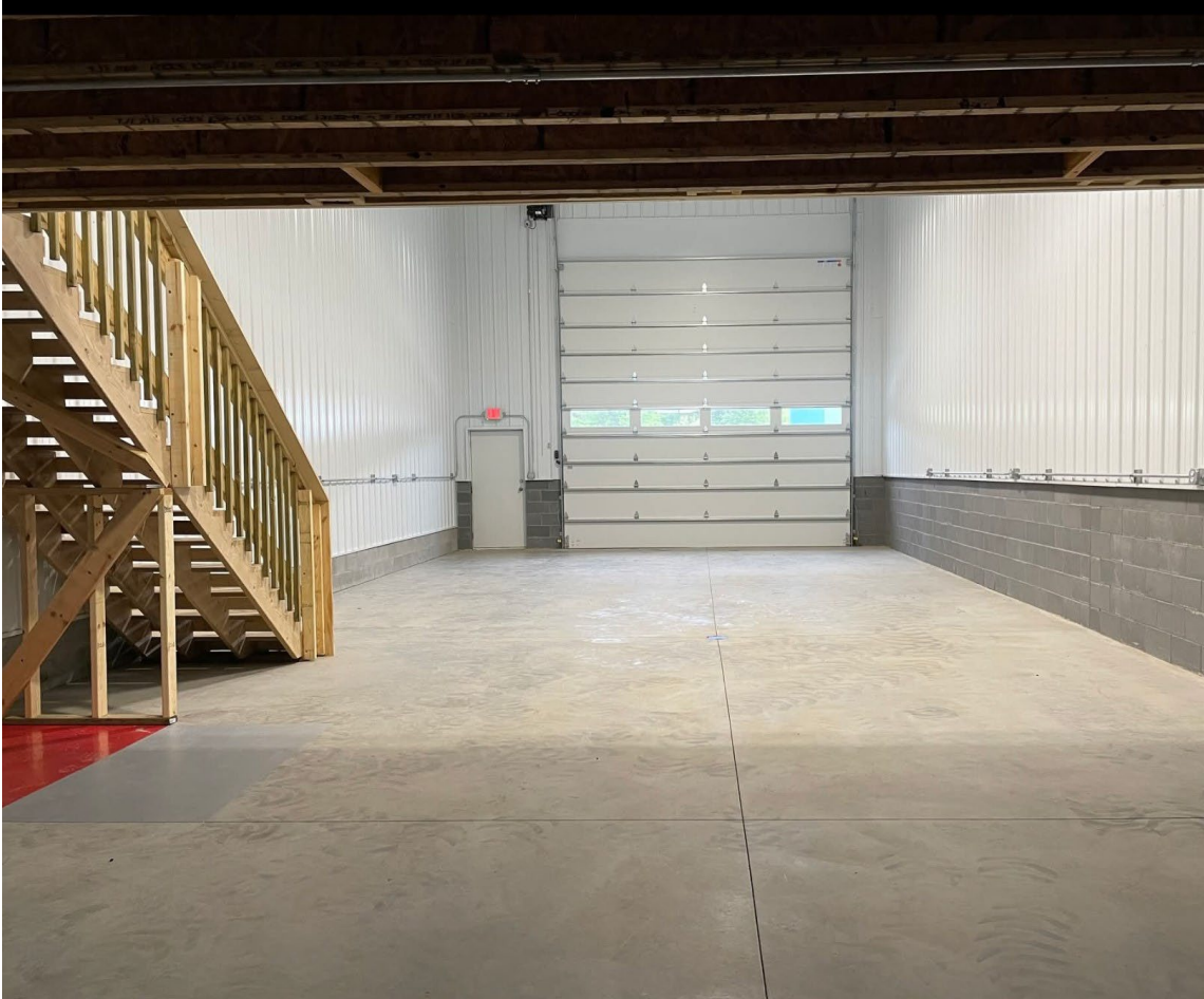
Clear-span interior storage unit
