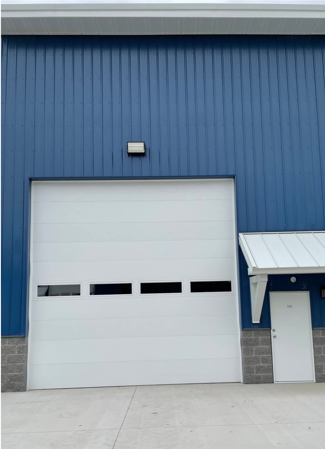
Unit doors and exterior lighting
