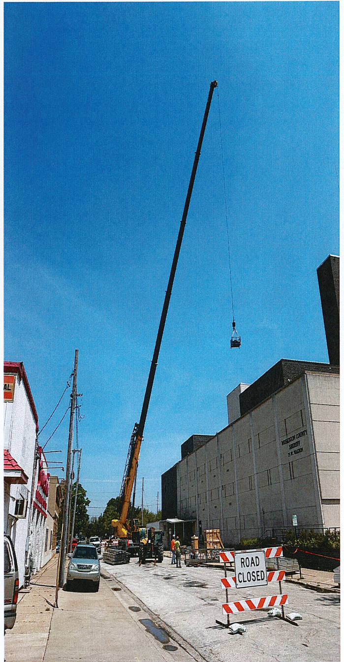
Crane lifting curtain wall material
