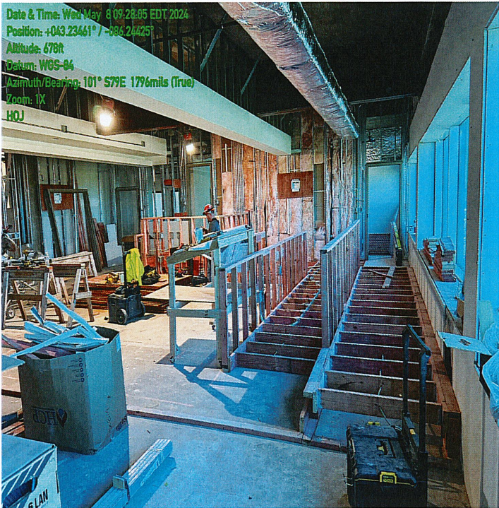
South courtroom under construction
