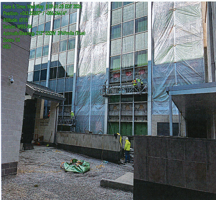
East curtain wall demolition
