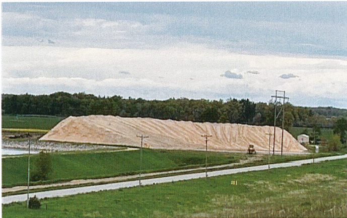
Sand stockpile for Cell 4/5 Final Cover project
